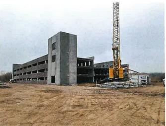
Parking Garage Erection – Interior (Elevator Tower Erected)
